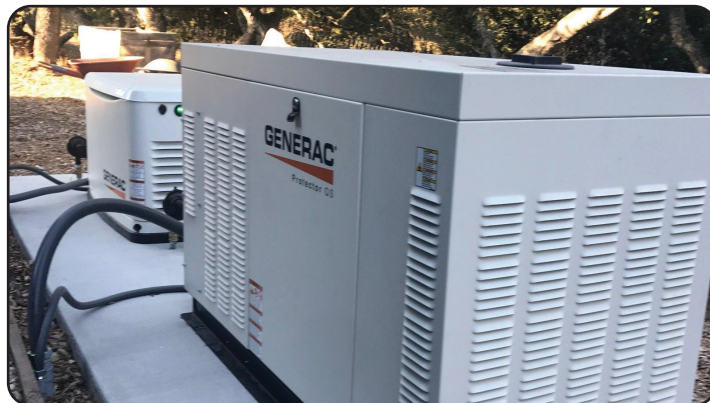
27 kilowatt liquid generac generator installed by Delta Liquid Energy
